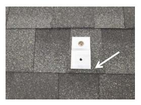
**4.** Base plate installed – note bottom edge of plate is 0.25" above shingle edge.
