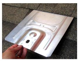
**7.** Slide flashing into position under shingle course above base plate.
