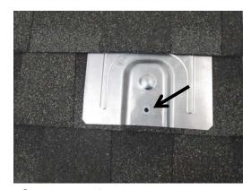
**8.** Align hole in flashing with threaded hole in base plate.
