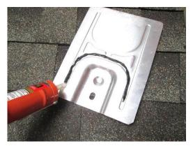
**6**. For maximum protection, sealant should be applied to trough in underside of flashing before installation.
