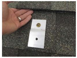
**5.** Lift shingle course above base plate slightly after loosening with roofing bar or similar tool to make room for flashing. Loosen just enough for flashing to slide up and under shingle (see photo, step 8).
