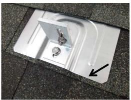
**10.** Completed flashing installation. Use T-Bolt and nut to secure racking to L-Foot. Note correct base plate/flashing position – edge of flashing is 0.25" above edge of shingle course. \*\*THIS ALIGNMENT IS CRITICAL FOR PROPER WATER-PROOFING\*\*
