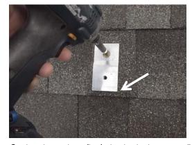
**2.** Place base plate, flat/ridged side down, 0.25" above shingle edge – note arrow in photo. Drive 4" fastener through unthreaded hole in base plate just far enough to confirm rafter location. This creates hole to accept roofing sealant.
