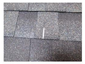
**1.** Mark location of rafters to be attached to as per engineering requirements. Determine which course of shingles is to be used for each row of flashings.
