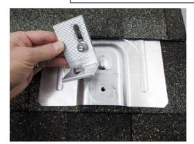
**9.** Attach L-Foot through flashing and into threaded hole in base plate using M8 bolt. Torque M8 bolt to 17-23Nm (13-17 Ft-Lbs)
