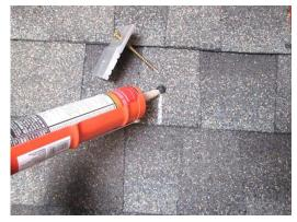
**3.** Fill hole with sealant then drive screw through *unthreaded* hole in base plate until snug. Do not over tighten – ensure base plate is flat/parallel to roof.
